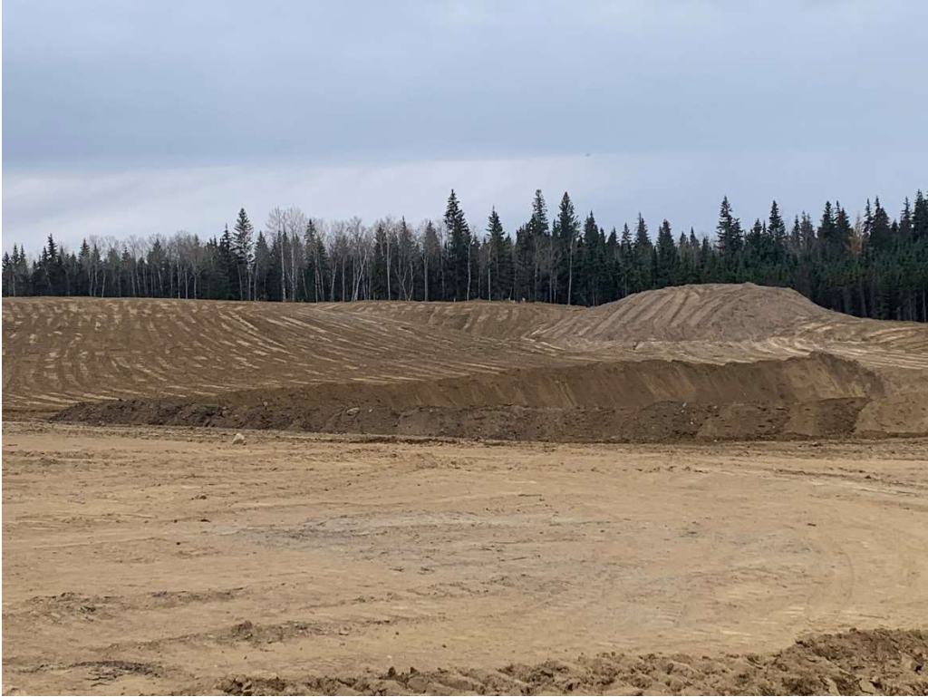
Photo 3: Photo looking south towards the hill utilized to backfill the waterbody.
