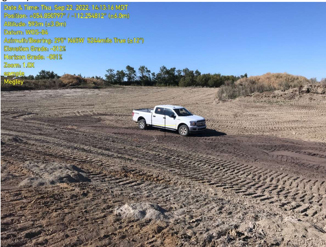
Photo 2: Photo taken looking northwest of the backfilling and recontouring of the dugout (2 nd waterbody on site).
