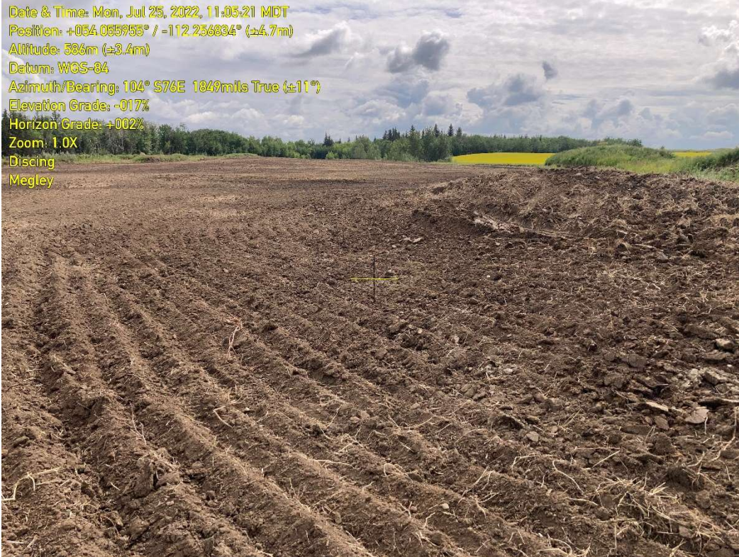
Photo 3: Photo taken looking northeast at the discing completed in the northern section of the pit.
